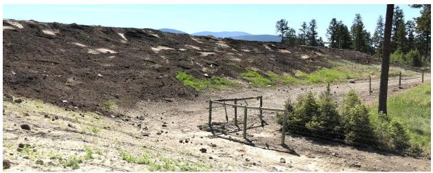
Photo 2. Slope 5 area west of current active cell received biocover in early 2018
