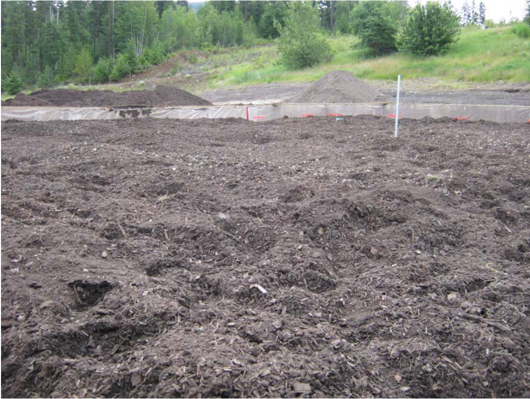
Figure 2. Clearwater biofilter surface before installation of the monitoring equipment.
