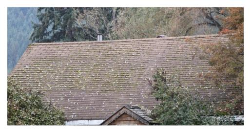
Figure 8 Aging roofs pose a potential risk to home ignition as the fire-resistant material begins to wear and expose a combustible underside
