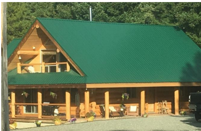
Figure 12 Fire-resistant roofing material provides excellent resiliency against home ignition. Simple roof designs can also contribute to the reduction of debris accumulation as pinch points are no longer a factor
