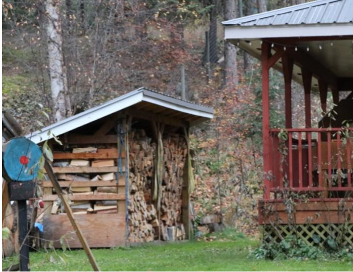
Figure 8 While this firewood has been offered some protection against ignition (i.e. firebrands from above) the continuous vegetation - grass - allows for fire to access the wood stack. With its proximity to the home (<10m) should the stack ignite it will very likely sustain enough radiant heat or produce enough firebrands to ignite the nearby structure.
