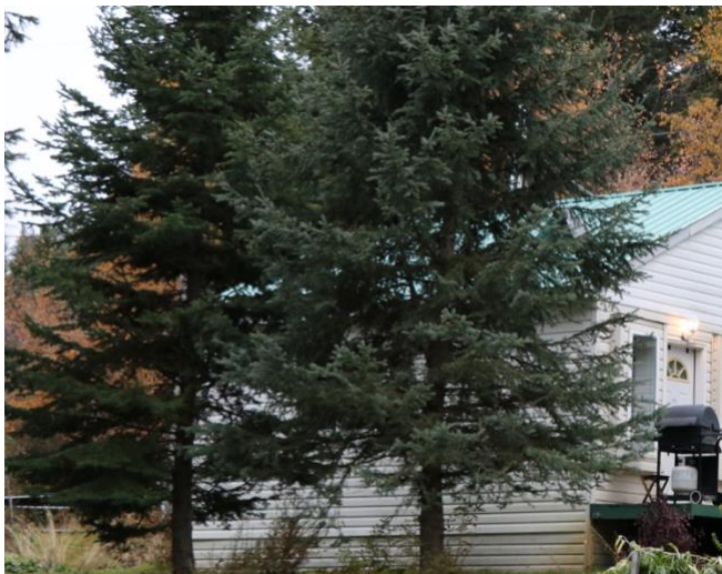
Figure 7 The presence of nearby combustible debris (such as wood pallets, ladders, building materials etc.) and combustible plants pose a high risk to ignition of a building's exterior
