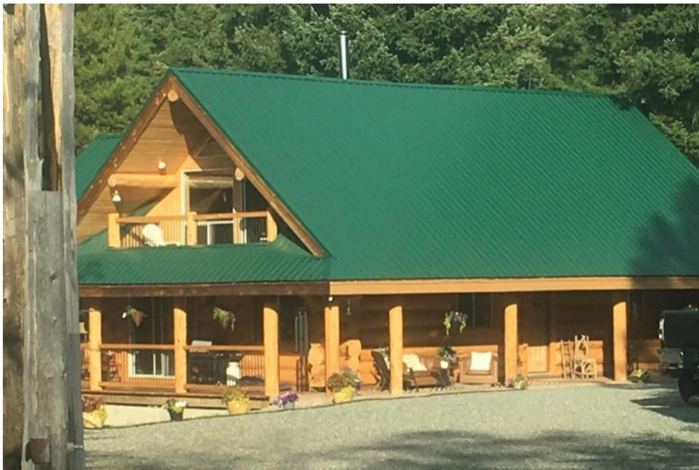
Figure 10 Fire-rated roofing material is proven to be highly resilient against home ignition during a wildfire event. Roof design can also contribute to mitigation of debris accumulation by minimizing valleys and pinch point where debris can be captured
