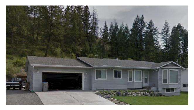
Figure 13 Concrete driveway, walkway and gravel help to disconnect the home from potential direct flame contact. Grass is kept green and at low growth therefore reducing the likelihood of intense burning. All other vegetation is kept 10m away from the structure.
