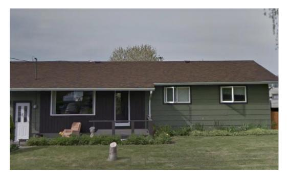
Figure 12 Fire rated roofing materials - asphalt, metal or clay - in combination with being free of debris provide increased resiliency against ignition from a wildfire
