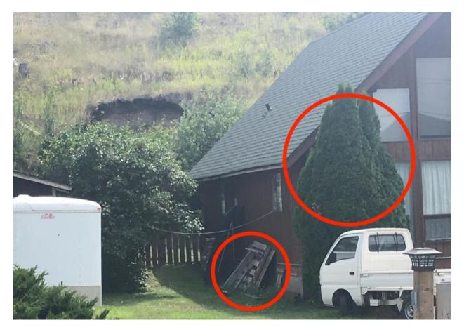
Figure 7 The presence of nearby combustible debris (such as wood pallets, ladders, building materials etc.) and combustible plants pose a high risk to ignition of a building's exterior. Vinyl siding was the predominant building exterior within the community. This material is highly susceptible to melting and sluffing from extreme radiant heat.
