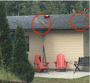
Figure 9 Debris accumulation on roofs is a potential ignition source that can decrease the fire resistance
