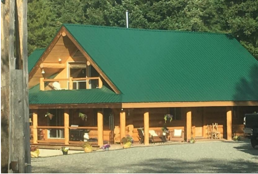
Figure 12 Fire-rated roofing material is proven to be highly resilient against home ignition during a wildfire event. Roof design can also contribute to mitigation of debris accumulation by minimizing valleys and pinch point where debris can be captured
