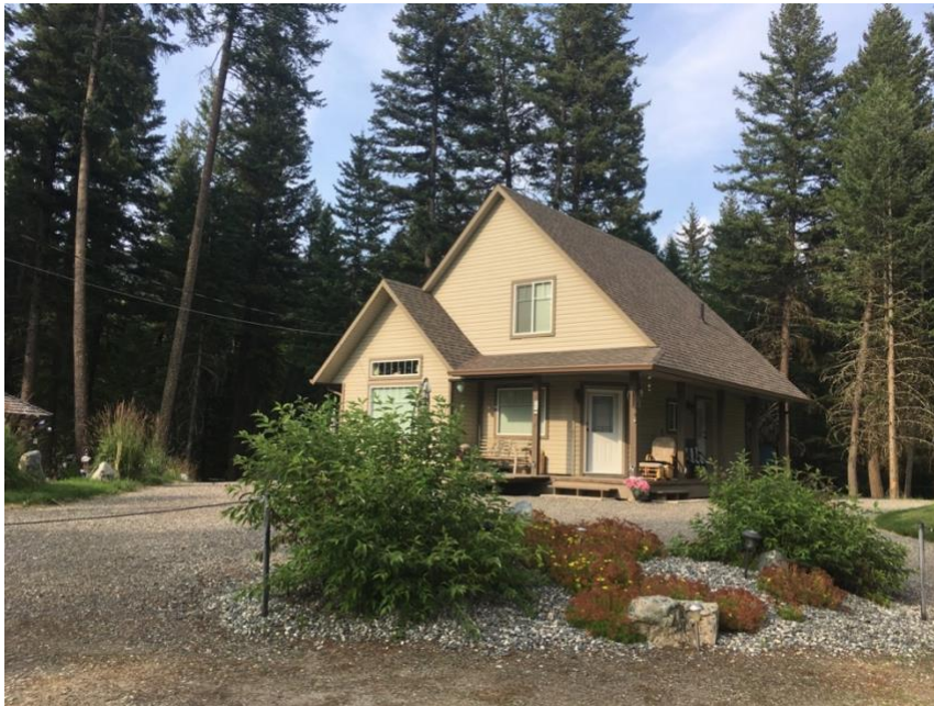
Figure 13 This home demonstrates several FireSmart landscaping attributes. The gravel provides a non-combustible surface creating a break from direct flame contact to the home. Conifers have been removed up to 10m away and ladder fuels have been cleared. Leafy, deciduous plants are the preferred vegetation to be found in zone 1.
