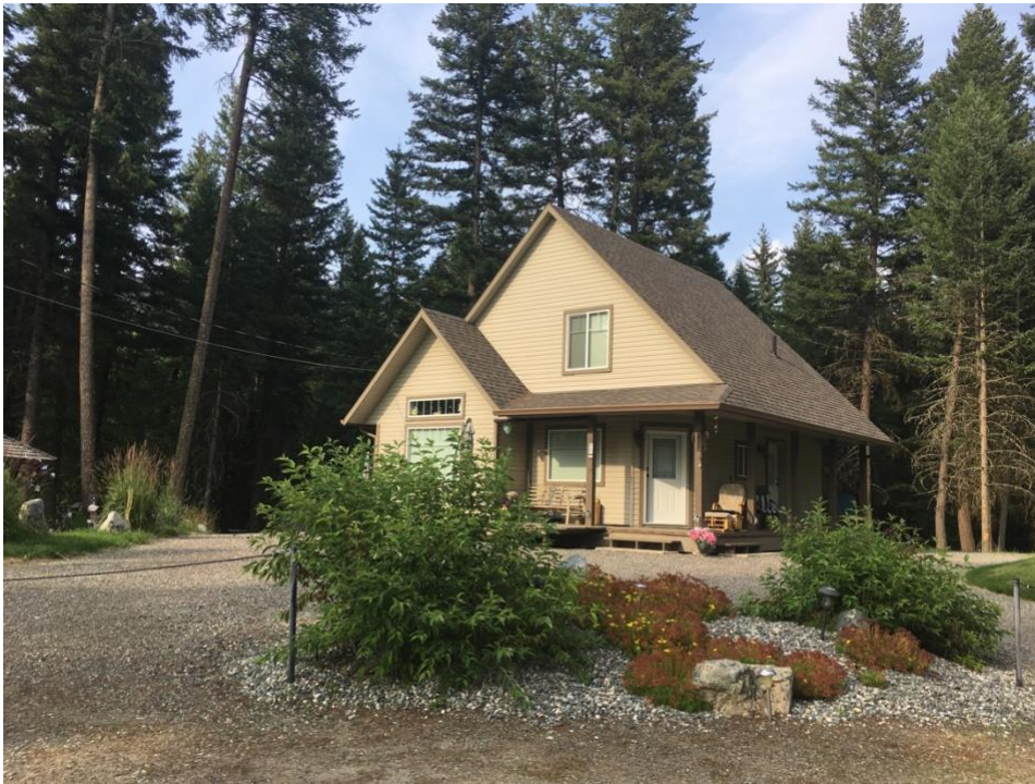
Figure 10 This home demonstrates several FireSmart landscaping attributes. The gravel provides a non-combustible surface creating a break from direct flame contact to the home. Conifers have been removed up to 10m away and ladder fuels have been cleared. Leafy, deciduous plants are the preferred vegetation to be found in zone 1.
