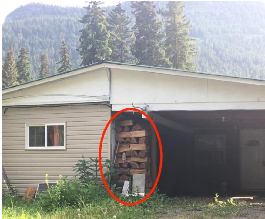
Figure 7 Firewood is a high-risk hazard for home ignition during a wildfire event. Firewood should be stacked a min. 10m away from the home during high threat of wildfire
