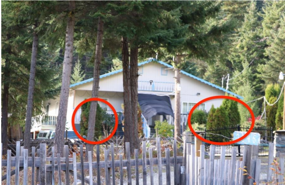
Figure 8 The presence of nearby combustible debris (such as wood pallets, ladders, building materials etc.) and combustible plants pose a high risk to ignition of a building's exterior.
