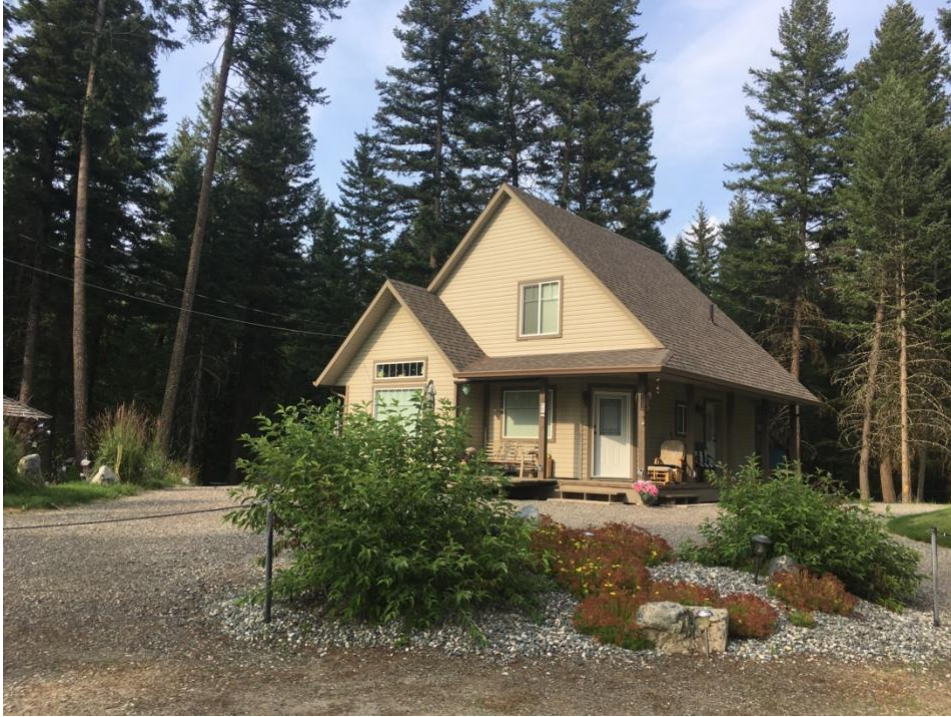
Figure 12 This home demonstrates several FireSmart landscaping attributes. The gravel provides a non-combustible surface creating a break from direct flame contact to the home. Conifers have been removed up to 10m away and ladder fuels have been cleared. Leafy, deciduous plants are the preferred vegetation to be found in zone 1.
