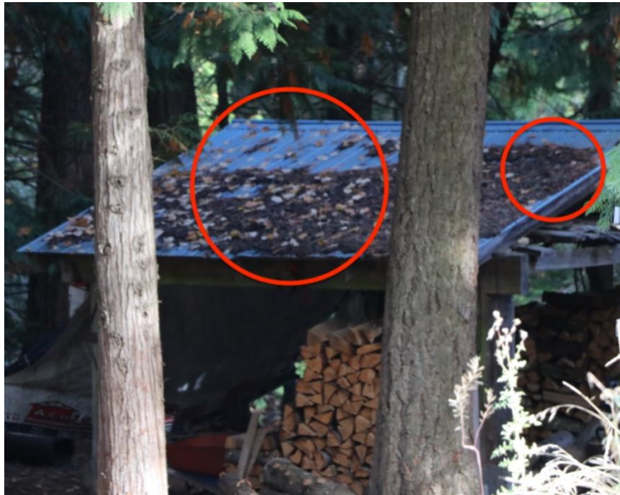
Figure 7 Combustible debris that ignites on a roof poses a risk of challenging a roof's fire resistance. As well, it has the risk to ignite other fuel sources (i.e. on the ground below) resulting in the spread of wildfire around a home.
