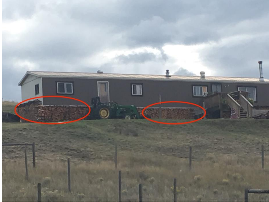
Figure 9 Firewood should be relocated >10m away from the home during times of high threat of wildfire
