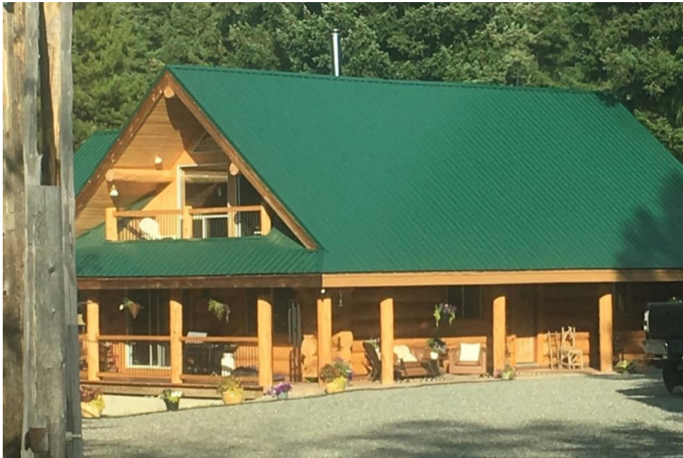
Figure 13 Fire-rated roofing material is proven to be highly resilient against home ignition during a wildfire event. Roof design can also contribute to mitigation of debris accumulation by minimizing valleys and pinch point where debris can be captured
