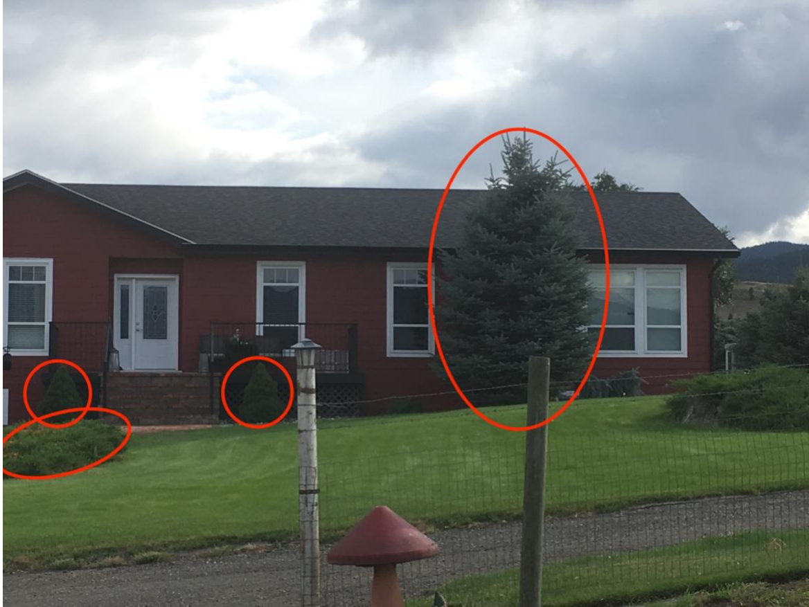
Figure 8 The presence of nearby combustible debris (such as wood pallets, ladders, building materials etc.) and combustible plants pose a high risk to ignition of a building's exterior.
