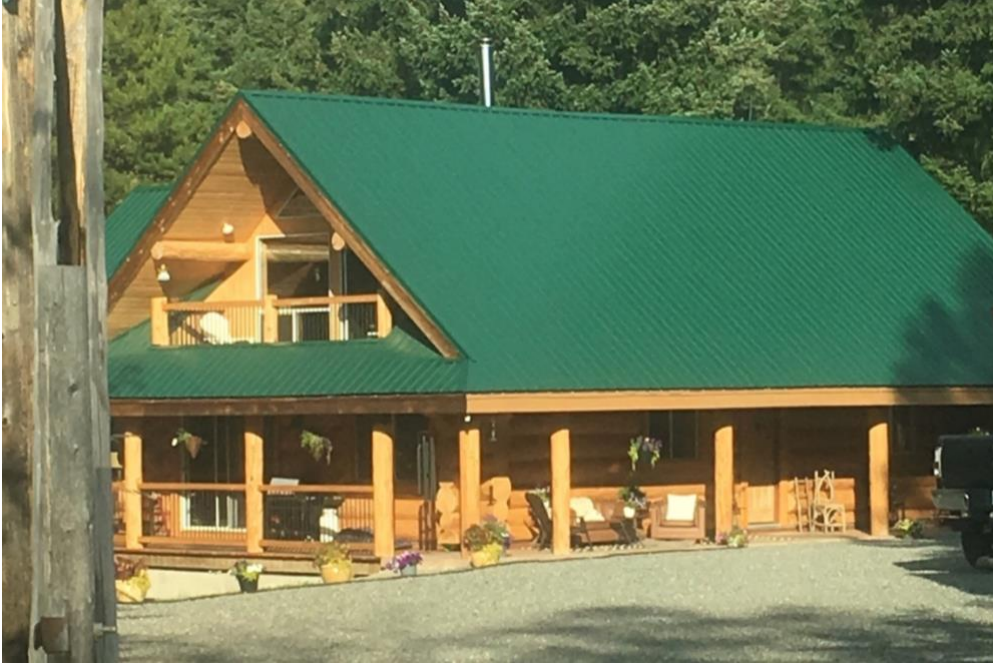
Figure 11 Fire-rated roofing material is proven to be highly resilient against home ignition during a wildfire event. Roof design can also contribute to mitigation of debris accumulation by minimizing valleys and pinch point where debris can be captured
