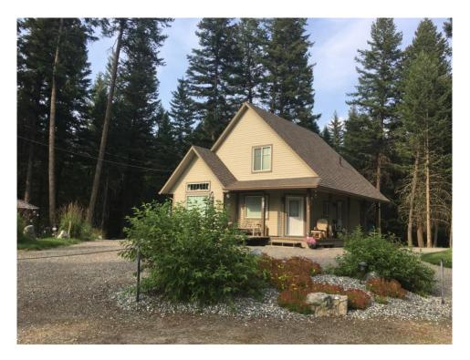
Figure 12 This home demonstrates several FireSmart landscaping attributes. The gravel provides a non-combustible surface creating a break from direct flame contact to the home. Conifers have been removed up to 10m away and ladder fuels have been cleared. Leafy, deciduous plants are the preferred vegetation to be found in zone 1.
