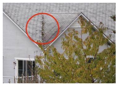
Figure 8 Combustible debris poses a risk to home ignition as burning debris can challenge a roof's resiliency to fire.
