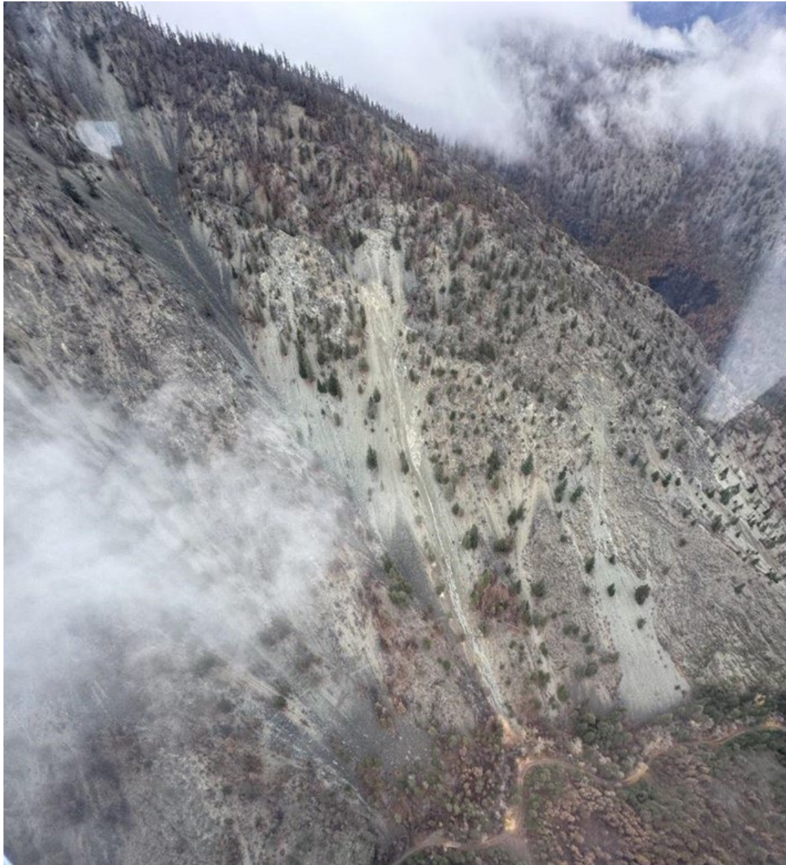
Photo D-38 Aerial-oblique photo of Murray Creek Rd and one of the three bridge crossings. Note the high relief and high sediment supply above the road.
