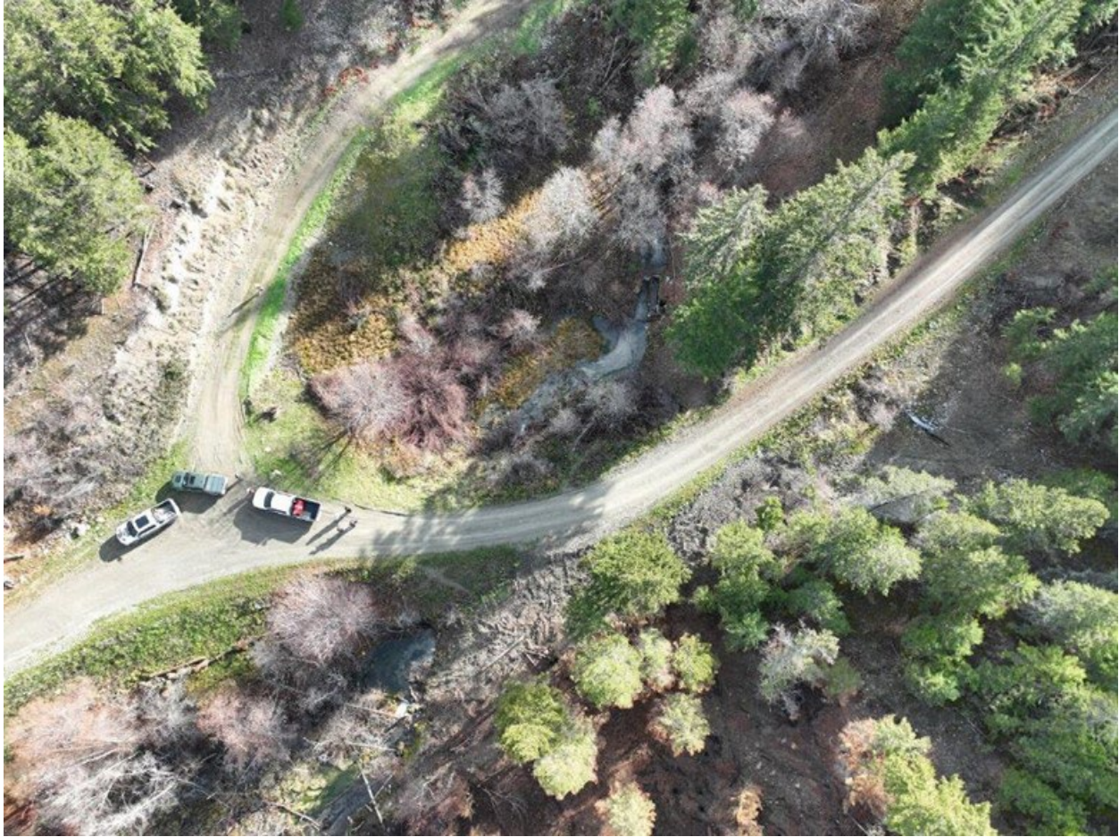
Photo D-32 Aerial overview photo of PD45750 water intake structure along Twaal Creek (center-top). Photo taken by BGC on November 18, 2024.
